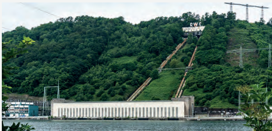
Koeppenwerk is one of the first large-scale pumped storage power plants to be built in Germany (1927–1930).
